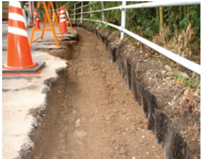
BambooBarrier™ installed
