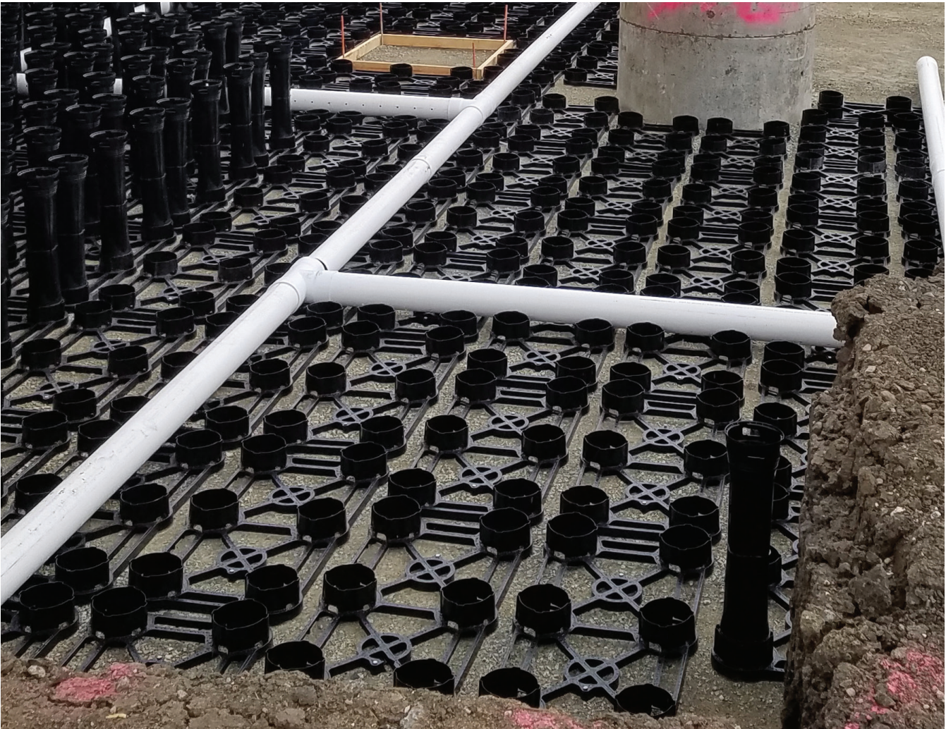
Above Underdrain being installed at base of system
