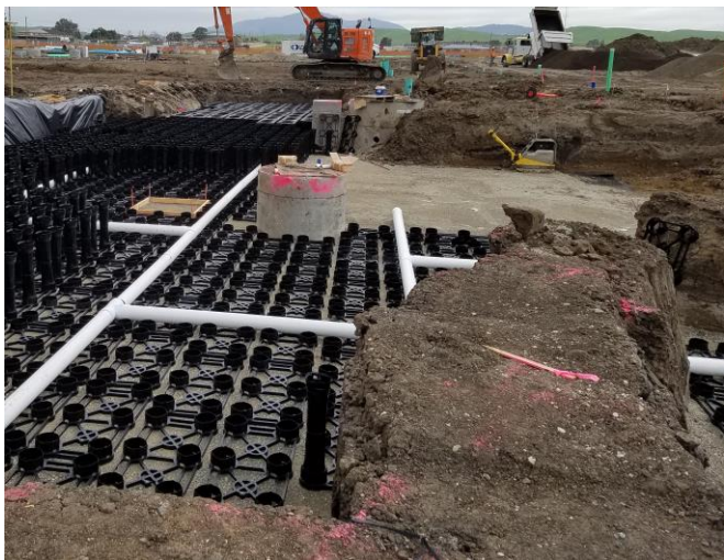
Underdrain being installed at base of system
