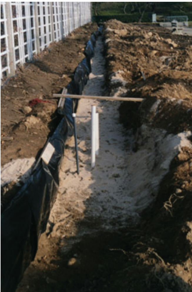
Damaged Multi-Use path
