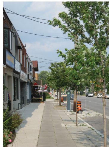
Asphalt covers the parking bay and pavers cover the sidewalk.
