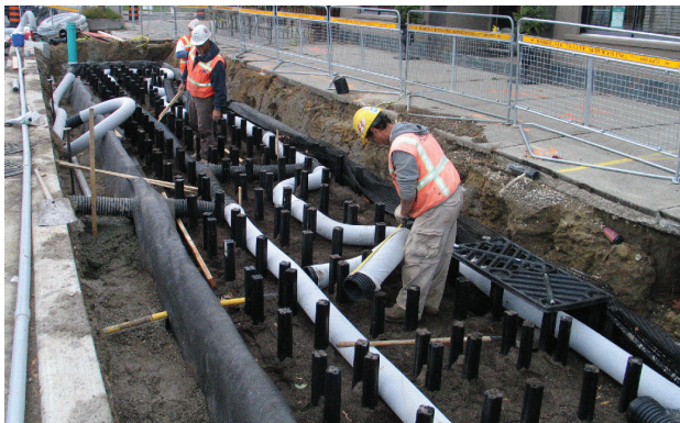
Perforated distribution pipes are placed throughout the system
