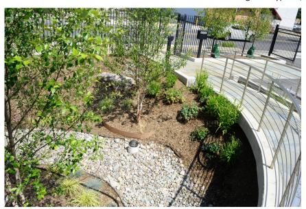
Both the District Department of the Environment (DDOE) and D.C. Water charge for water runoff by calculating impervious surface area on a property. However, property owners may mitigate these charges through green infrastructure solutions that capture and manage stormwater on-site. The Casey Trees head-quarters project showcases how keeping stormwater on-site can mitigate these charges while nourishing large urban tree growth.
